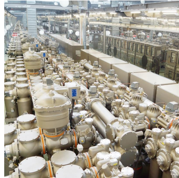
Eco-efficient Gas Insulated Switchgear
